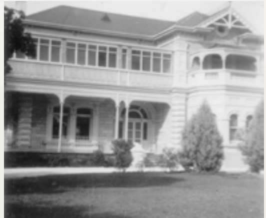
Fullarton Girls Home 2005 now the SA Divisional Headquarters of the Salvation Army, Courtesy Kay Goodman-Dodd. Fullarton Girls Home, Courtesy The Salvation Army Territorial Archives Melbourne
